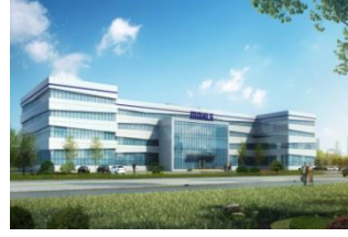
Under construction: the new R&D center in Suzhou/China, where components for Chinese e-mobility will be developed.
